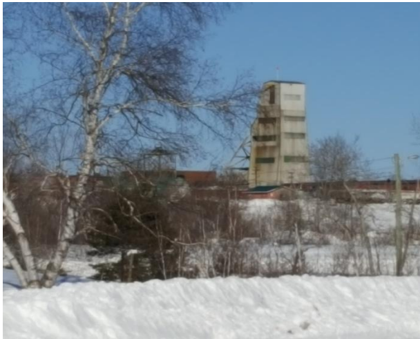
Garson Mine (Brown's boyhood home would have been just out of frame, to the right).
