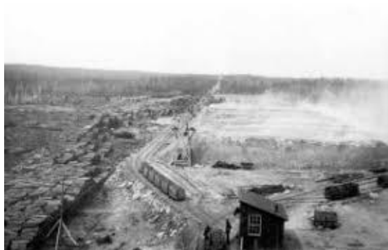
Open Ore Roasting Beds, Coniston ON, in the 1920s.
